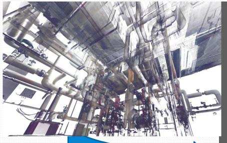
Feature recognition software takes the point cloud and identifies pipes, ductwork, walls, floors, doors and windows into parametric models.
